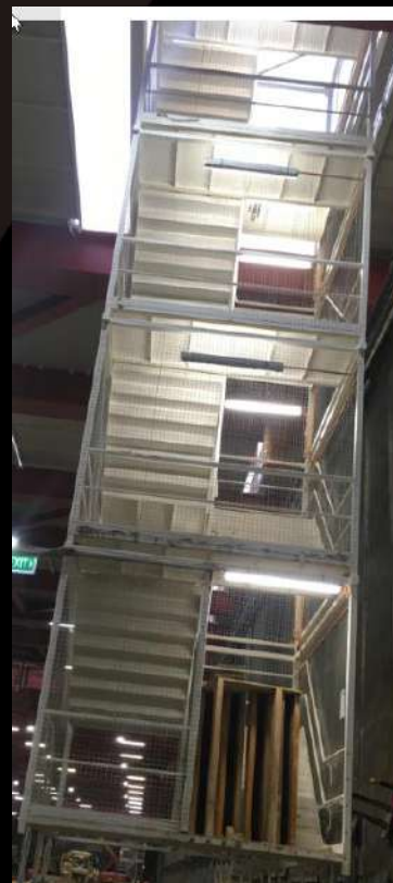
LANDING FRAME OVER GIRDER
