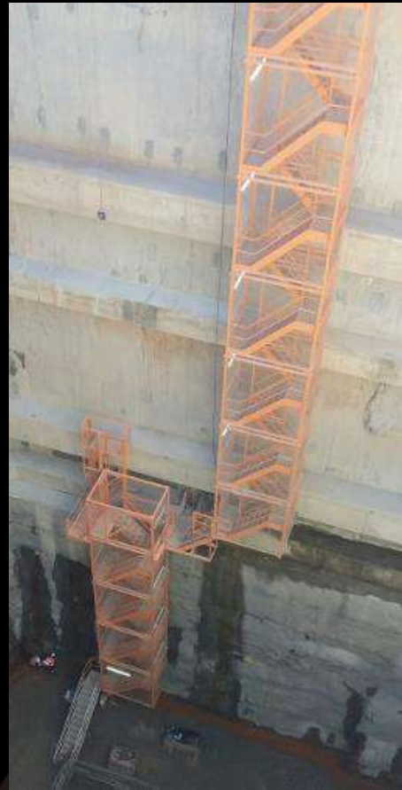
LANDING FRAME OVER GIRDER
