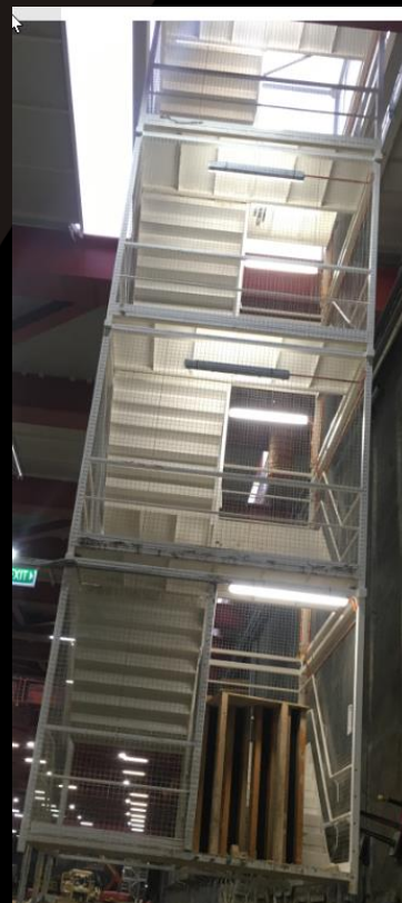
LANDING FRAME OVER GIRDER
