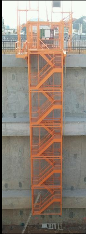
STAIR SYSTEM OFFSET FROM WALL
